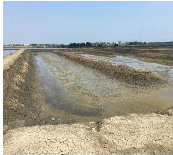
Fig.2 Maximum pond area is 0.32 hectare. Pond depth is 1.50 meters. Slope distance is 1.80 meters. Width is 2.50 meters.
