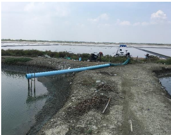
Fig.3 Pump seawater into the pond, water level is 1.5 meters.
