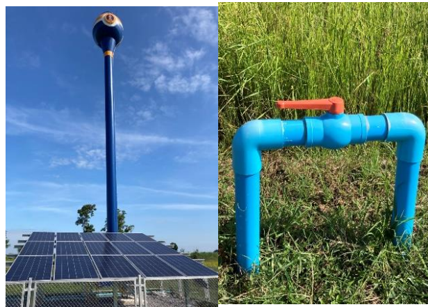
Fig. 8 The artesian well pumps water with solar cells together with the water distribution system supported by Department of Groundwater resources
